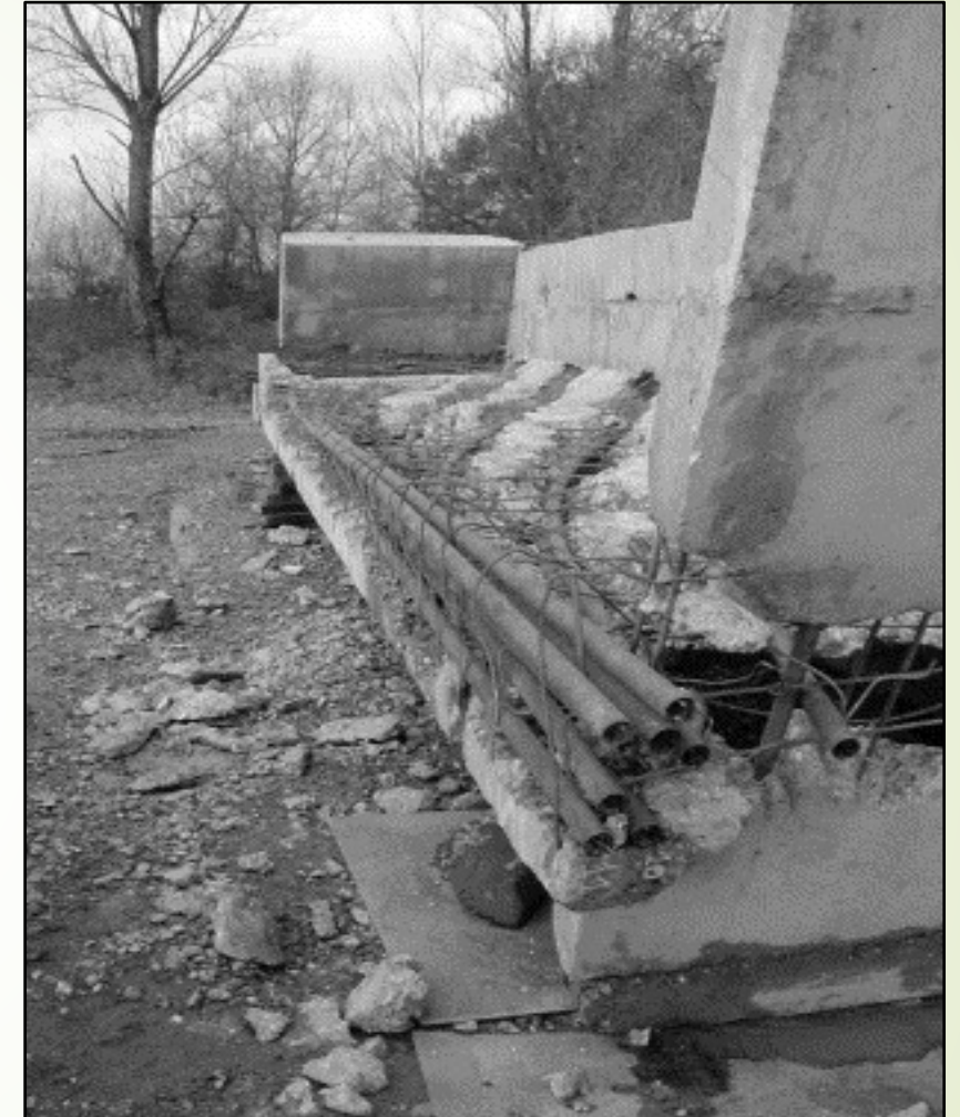
Release of tendons and anchorages from the beam after hydro-demolition
