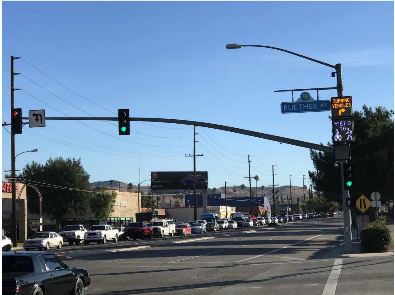
Blank-out signs to advise drivers of the presence of pedestrians or bicyclists entering the crosswalk.
