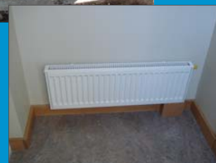
Standard low temperature radiators deliver comfortable heating in the Bauman-Broussard home.
