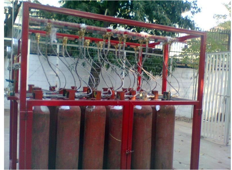
Bank of Hydrogen cylinders
