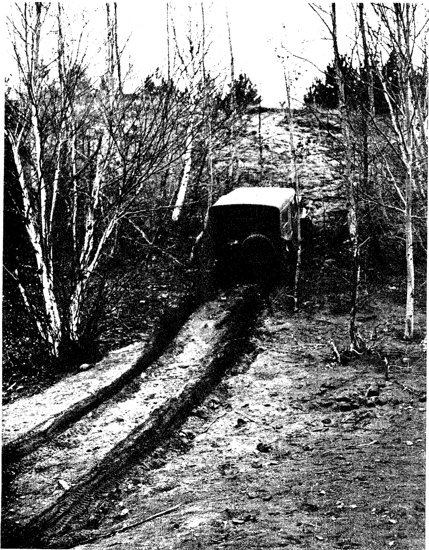
Figure 10A Gradeability Test on Packed Dirt
