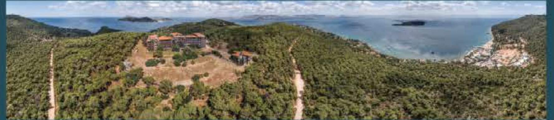
RUM YETİM HANESİ VE ÇEVRESİNİN HAVADAN GÖRÜŞÜ. 2018. (FOTOĞRAF: MURAT ÖZTİNK) AERIAL VIEW OF GREEK ORPHANAGE AND ITS SURROUNDINGS. 2018. (PHOTO: MURAT ÖZTİNK)
