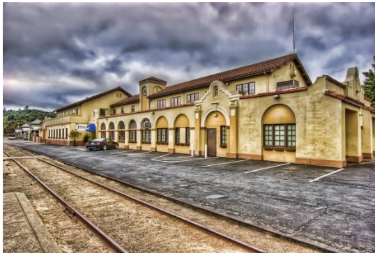
San Rafael's old train station – now being used by Whistlestop.
