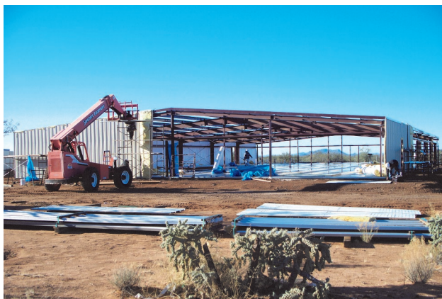
Apprentices of Carpentry and Facilities Maintenance are constructing the steel building with oversight by journeyman iron worker Marvin Enis.
