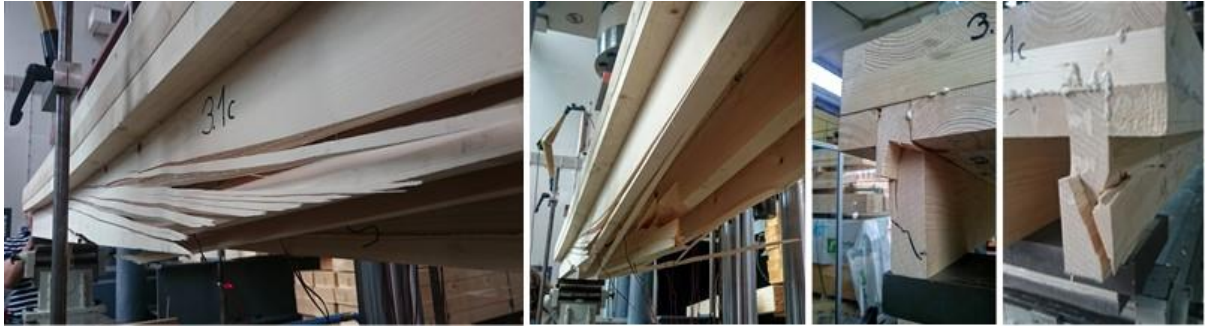
Figure 10: Damage in the XR-lam plates (either bending or shear) that occurs in several steps
