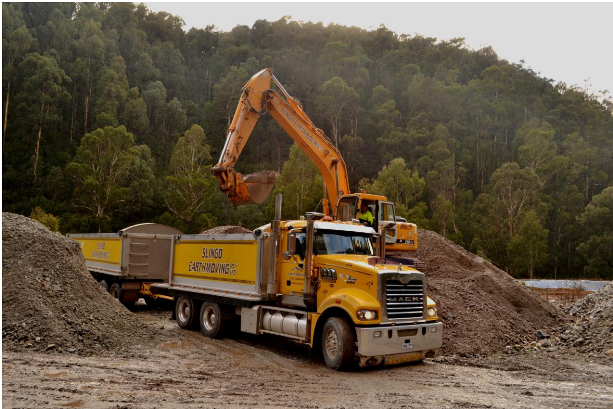
Figure 2. Loading of ore at A1 Mine ROM Pad
