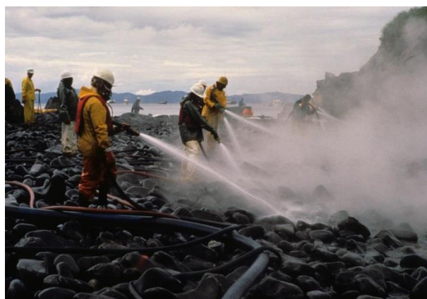
Fig. 11. A photo of high pressure flooding of oiled rocks
