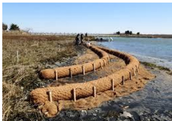
Fig. 9. A photo of shoreline barriers and berms (Source: https://www.google.bg/search? )
