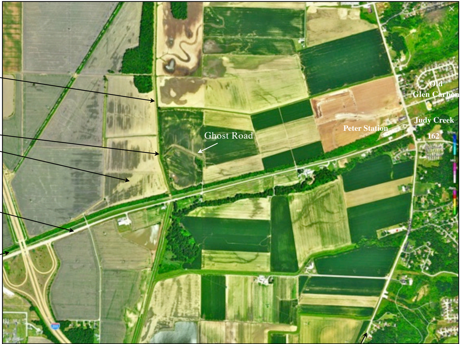
Aerial Photograph Showing the area where the original bridge built by D.D. Collins was located
