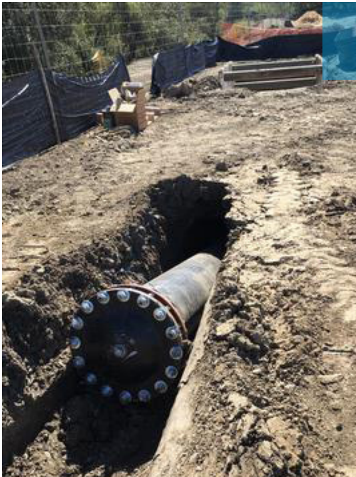
THE EXPOSED SECTION OF THE 18" HDPE PIPE THAT TRAVELS UNDERNEATH THE SALINAS RIVER.
