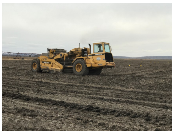
A scraper making a shallow water excavation on a former Missouri River oxbow site.
