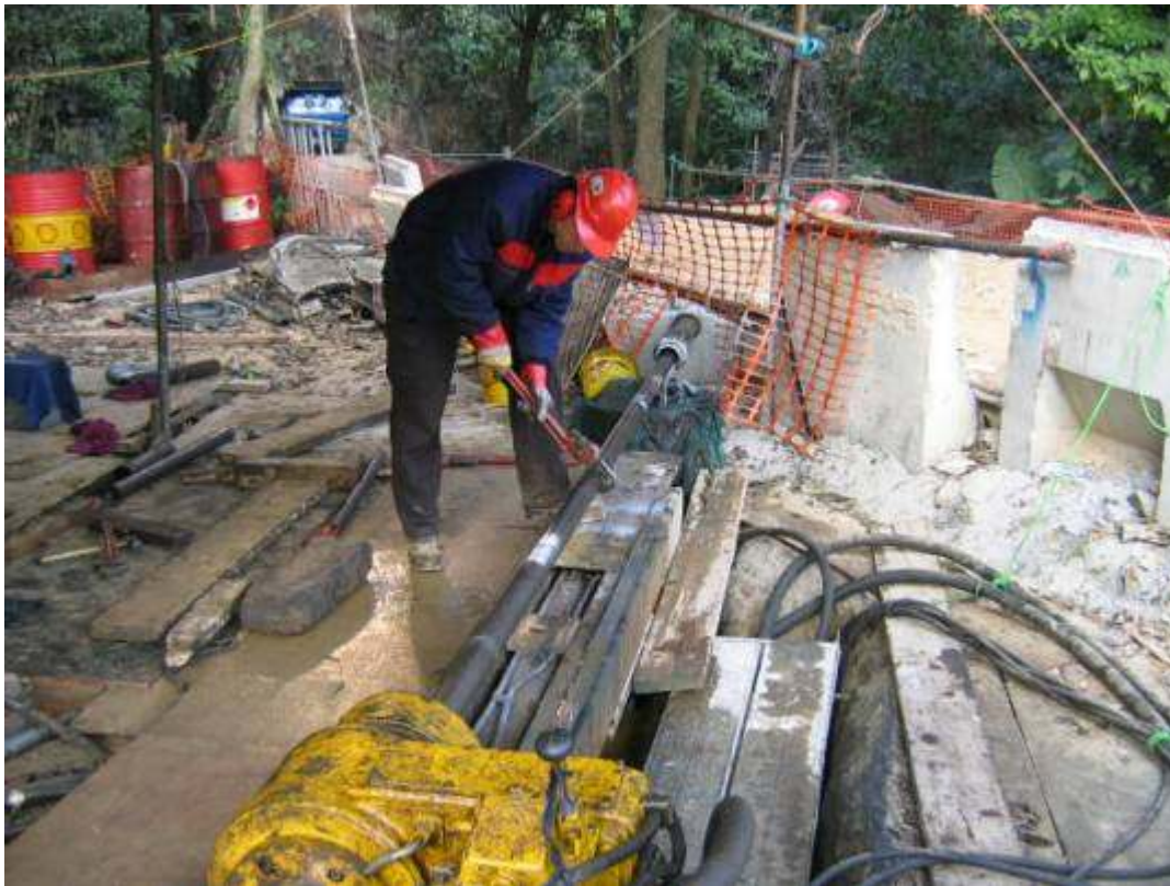
Adjusting the Toolface
