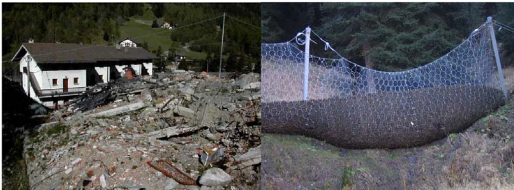
Figure 1: Debris flow deposit directly in front of a building and a filled flexible barrier system.
