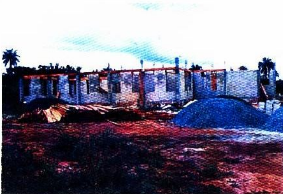
The Enterprenueral Building
