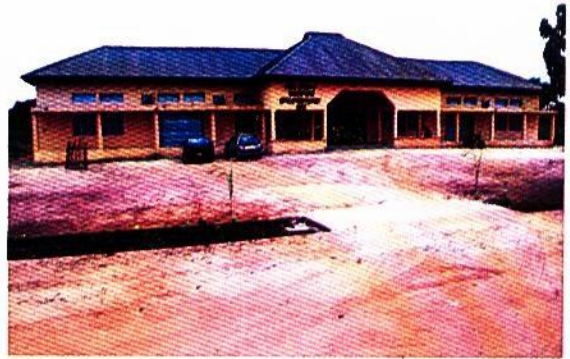
Central Instrument Equipment Centre
