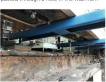
the inside to the outside. Prop Pal is designed so that a builder's prop location into the needle is locked into position once it has been wound up. At the other end the swivel plate has four holes allowing it to be fixed to the floor boards securing its position. It has been proof tested to a safe load capacity of 1,500kg.
