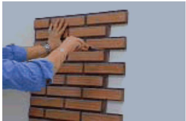
We drill in the wall with a drill of 6 or 8 mm right in the places where we have marked previously and we introduce 6 or 8 mm wall plugs. Screw into the wall until flush
