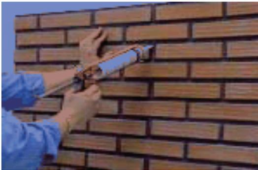
Once all panels have been fixed on the wall, use the mastic filler and apply it with the help of a application gun and a fine brush (to texture the mastic). All joints and drill holes must be filled.
