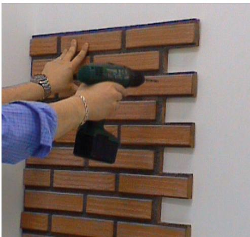
We place the panel on the wall and we drill across the panel marking on the wall with a 3mm drill. 4 to 8 holes per panel would be needed. Preferably in the cavities between the bricks
