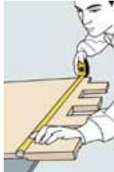
Measure the surface to make sure covered and calculate how many panels will be needed. Each one is approx. one square meter.
