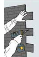
Place the panel on the wall and use the 3mm bit to drill through the joints across the panel till you get to mark the wall where wall plugs will be fixed later.
