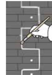
Then texture joints using a wet thin paintbrush
