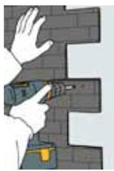
Place the panel on the wall and insert screws in the holes 2-3mm into the panel so we can then hide them with the putty
