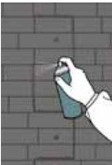
The spray is used to balance colours between joints and panels. So once the paint is dry spray over the joints one flash at a 40cm distance
