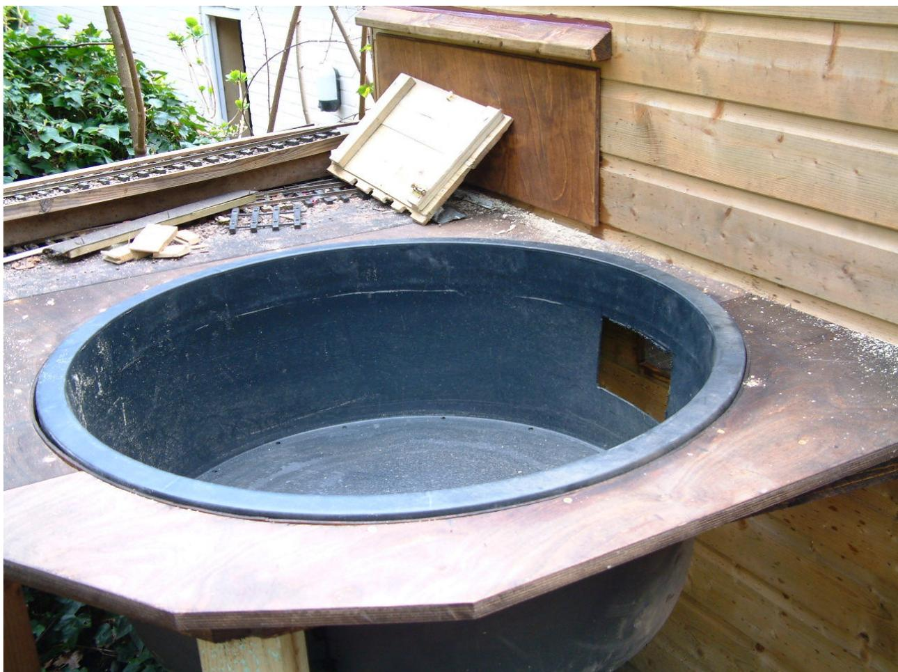
The benchwork was designed to allow the tank to be supported with the rim flush with the bench top, allowing plenty of depth for the 3½ inch clearance required for the rotating bridge and for the turning mechanism beneath the deck. For the latter one needs a sheet of weatherproof and stable material which must also be strong enough to mount a bearing for the central pin and also to sup-
