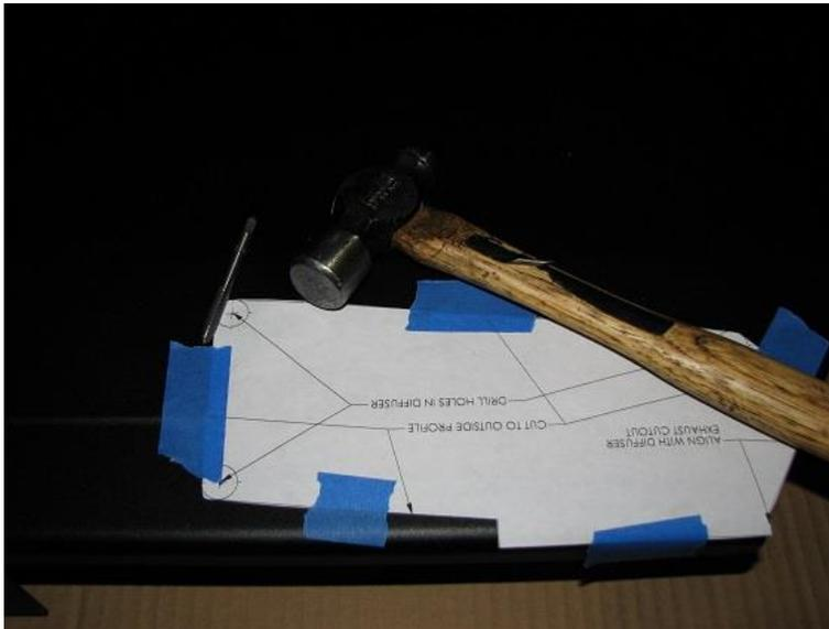
6.6. With these holes center punched, use the pilot drill bit to get the holes started.
