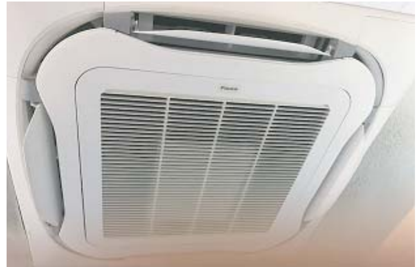
Air-con unit with Tera-Net (White Net at the center)
