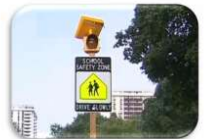
Flashing Beacon with Timer
