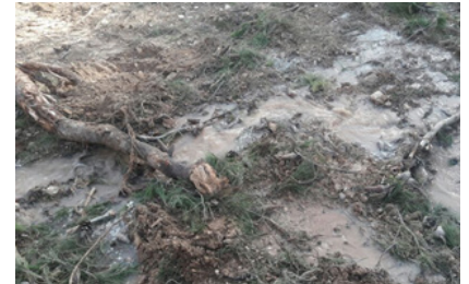
Eventually, the main leak was found in a natural creek outside the residential area. Without TaKaDu, the leak would probably not have been discovered for another 6-10 months.
