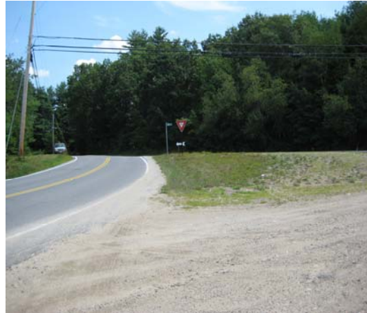
Eastbound Scribner Road Approach to Gile Road- Confusing Signage and Evidence of Use of Shoulder for Turns
