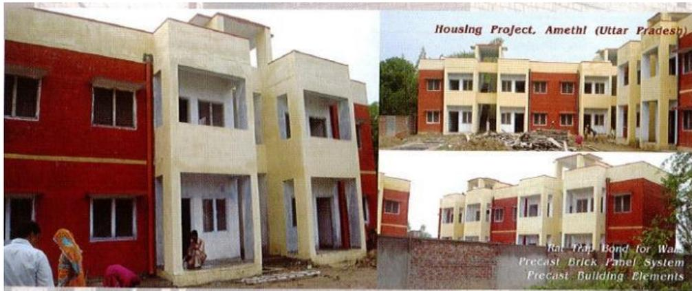
LIG housing in Uttar Pradesh - using Rat-trap bond walls and Precast brick panel system
