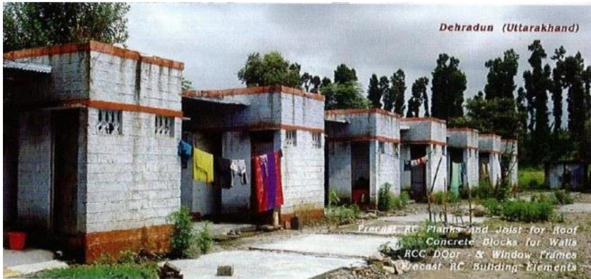
EWS housing in Dehradun, using Concrete Blocks, Precast RCC Planks and Joists and RCC door-window frames
