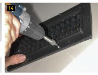
[13 and 14] The Fabulous Range Hood Upgrade Kit utilizes a gasket on the exterior vent, eliminating the need for butyl tape. Do not overtighten the screws, as damage to the plastic may occur.
