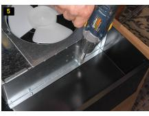
[4] Removing a single screw that holds the tin box in place exposes all of the wiring needed for modification. [5] Remove the four screws holding the original fan box assembly in place and set them aside for reinstallation; discard the box assembly. [6 and 7] Depending on the model of the stove exhaust vent assembly, one or two tabs may need to be straightened to remove the fan assembly.
