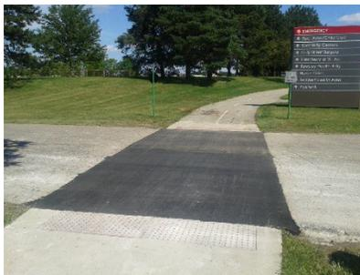
In July, B2B road crossings around St. Joseph hospital in Ypsilanti were repaved, making these crossings much more smooth and safe. The previous pavement had deteriorated to the point where cracks and crevices could catch a bicycle tire. The photos show the trail before and after the repaving.
