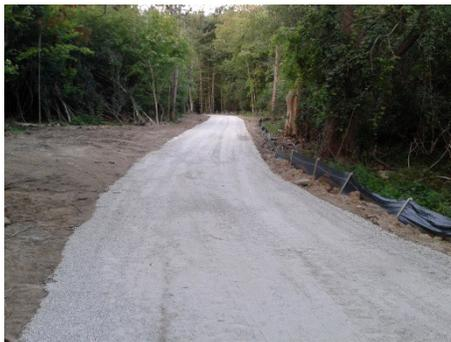
As of early August, construction of this new trail from the northeast corner of Geddes and Dixboro Roads north to the University of Michigan Matthaei Botanical Gardens was making solid progress, with a stone base constructed in preparation for paving with asphalt. Expectations are that the trail will be ready for use in the early fall. The Dixboro Trail connects to the B2B via existing trail through Parker Mill County Park.
