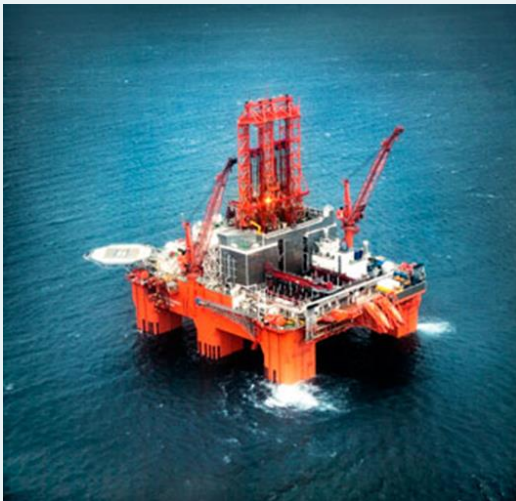
The West Phoenix semi-submersible rig.
