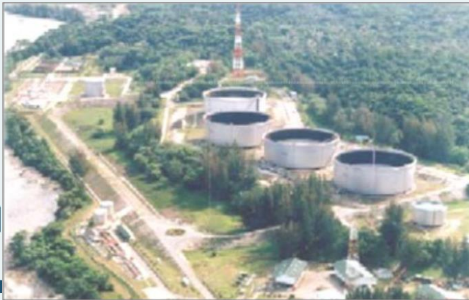
Labuan Crude Oil Terminal
