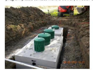
Picture to the left is an aeration tank and dosing chamber for a household sewage treatment system.
