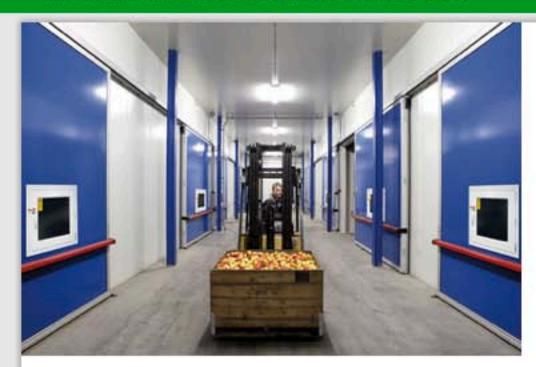
Door leaf constructed of a core of 100mm insulation material, covered on both sides with polyester and finished all round with anodized aluminium profiles, thermal bridge-free. Equipped with an aluminium drop/lift rail
