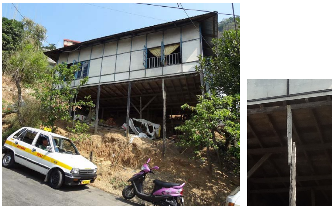
Figure 1. A traditional timber Assam-type building on an active landslide in Ramthar Veng (left) showing an inadequately braced natural timber post support system that accommodates the slope; a tenuous splice connection in a vertical support post in the same structure (right)
