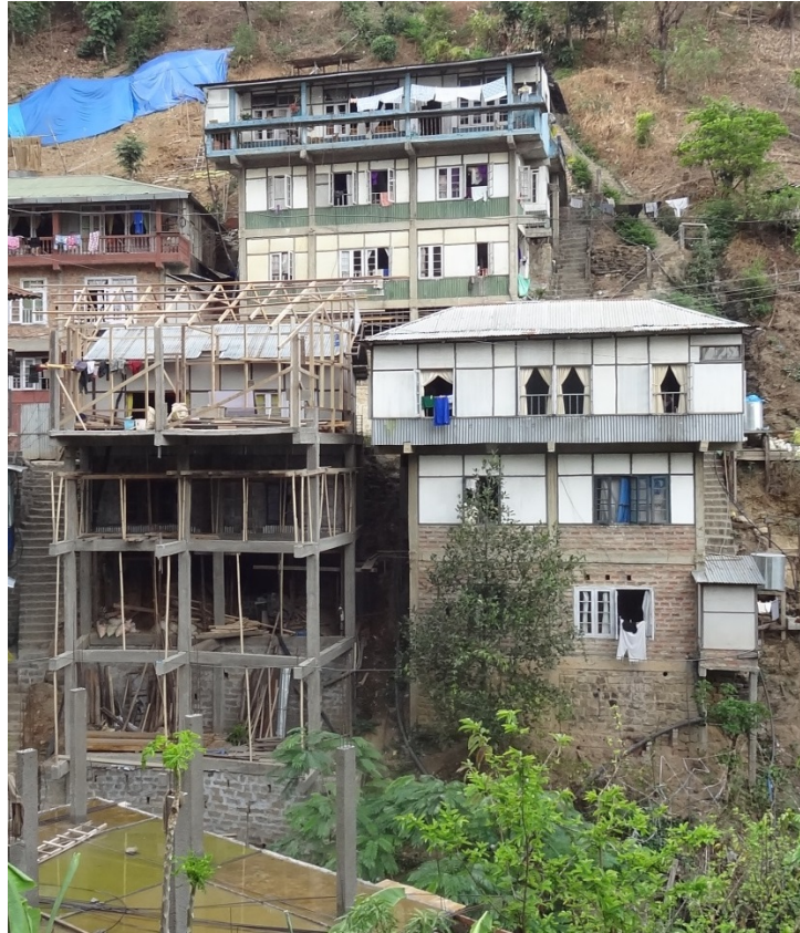
Figure 2. Semi-pucca buildings in southeast Aizawl; note concrete slab at top level of building under construction and lightweight walls that have been replaced by brick in building on right.
