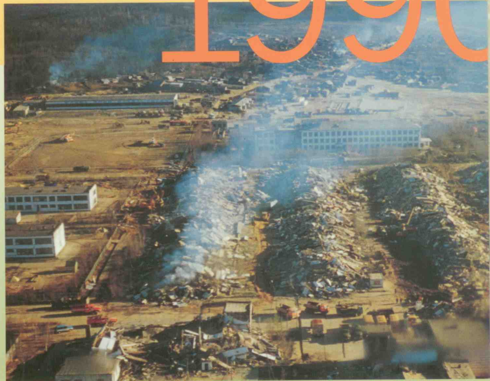
The quality of building construction in Central Asia today is similar to that found throughout the former Soviet Union, including the Russian city of Neftegorsk, pictured in this photo hours after an earthquake in 1995. The remains of these five-story residential structures, shown here as they fell, lie among damaged but still standing structures of different types.
